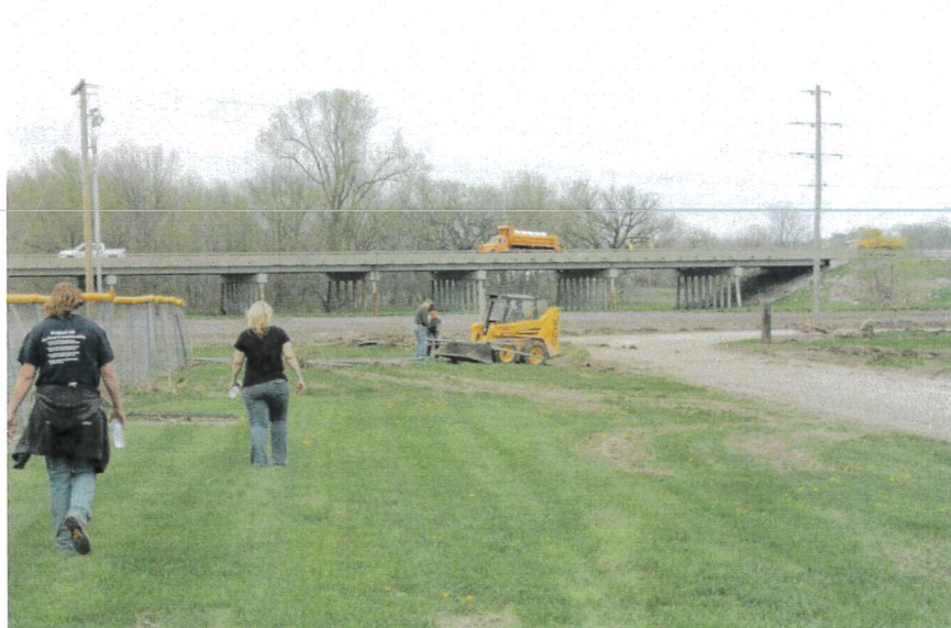
Volunteers work to fix fence after river currents cause damage to the ball fields. (2013)
