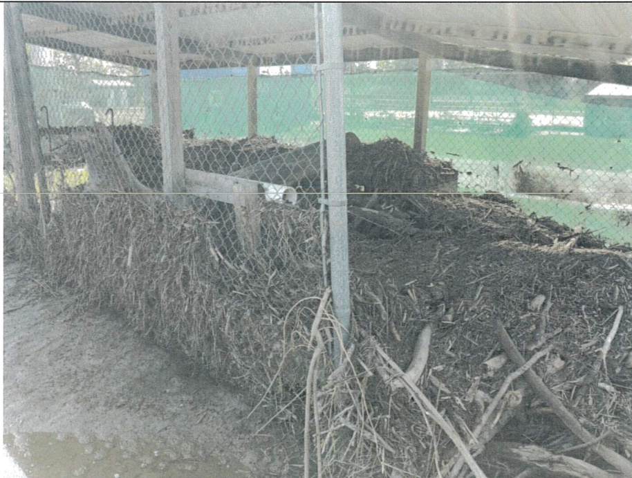
Debris from the river current destroys fences and results in loss of opportunities for the community. (2019)
