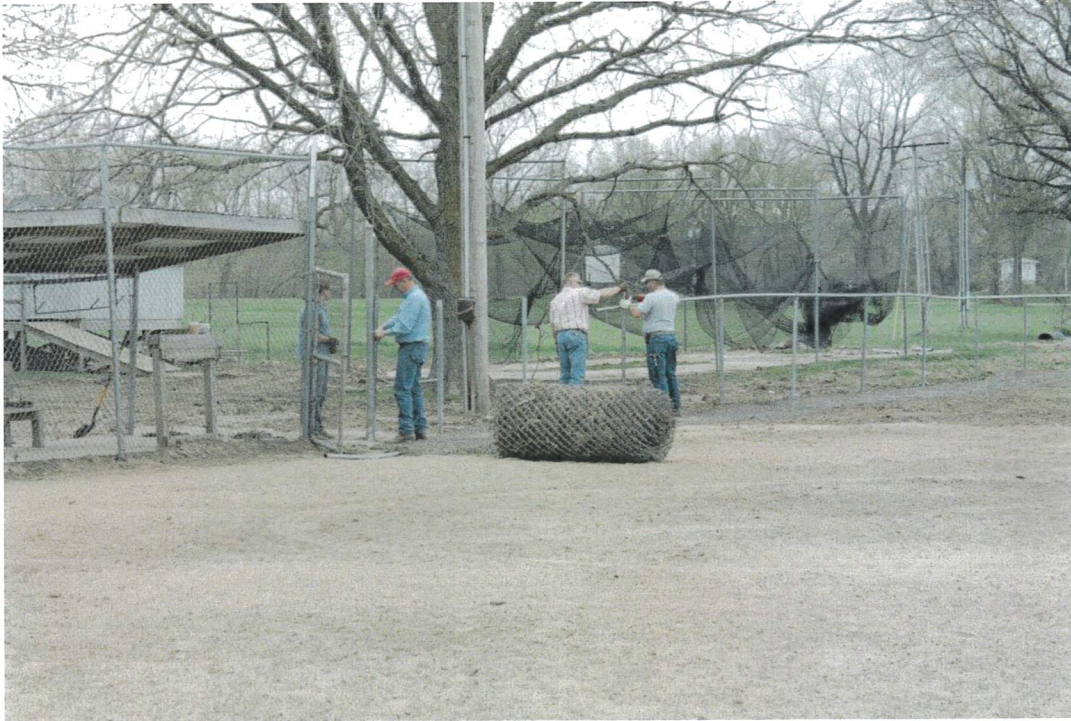
Volunteer work to replace damaged fence after flooding. (2013)
