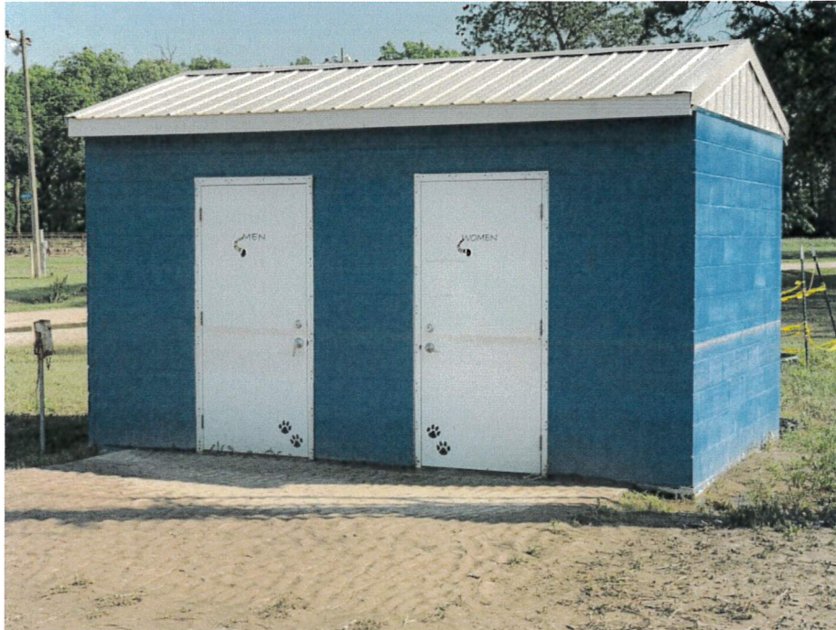
Floodwater level shown at the restrooms located at the existing ball fields. Flood waters cause major damage to the septic tanks and cause pollution to the river waters. (2019)
